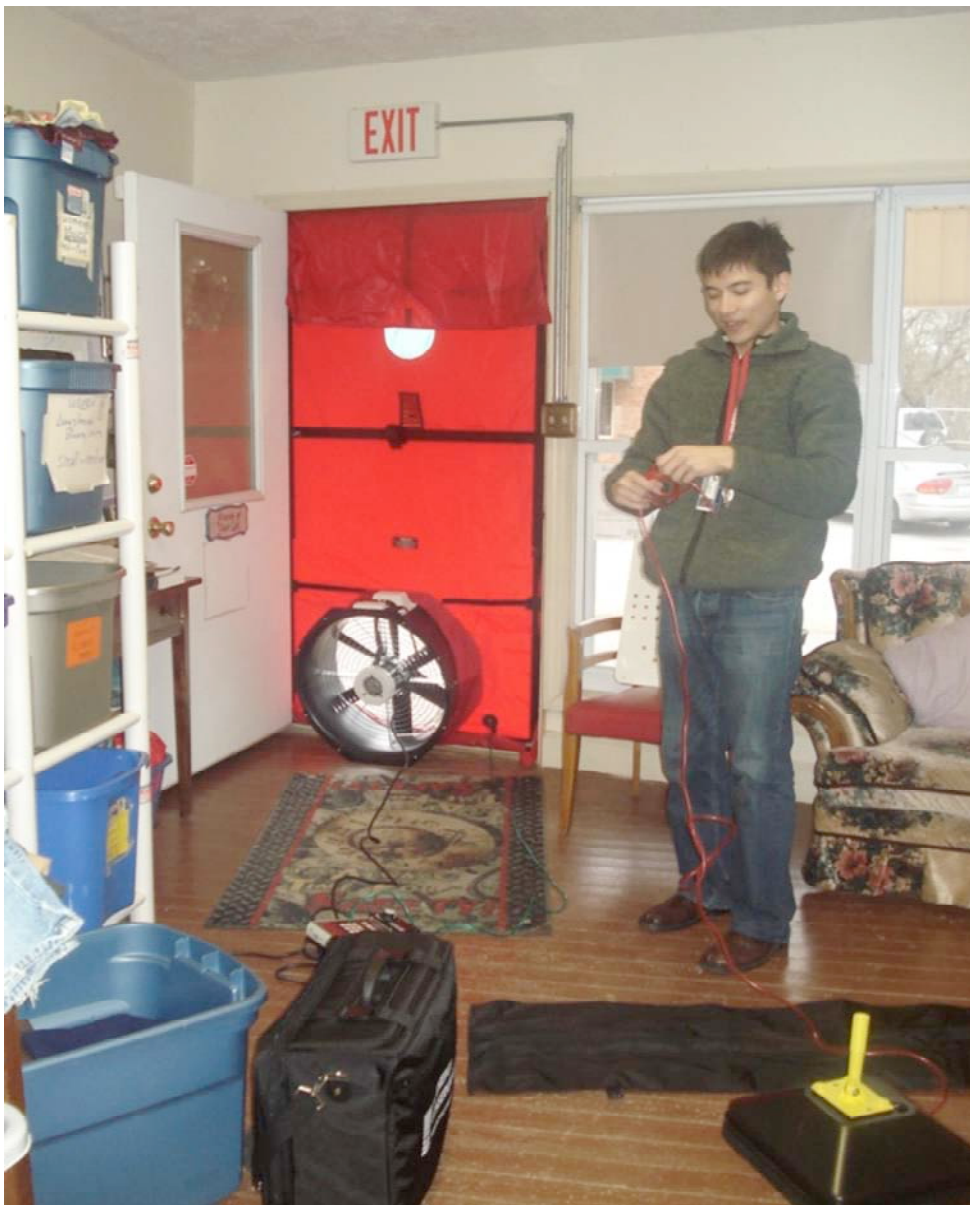
Blower door test photo courtesy of MACED
