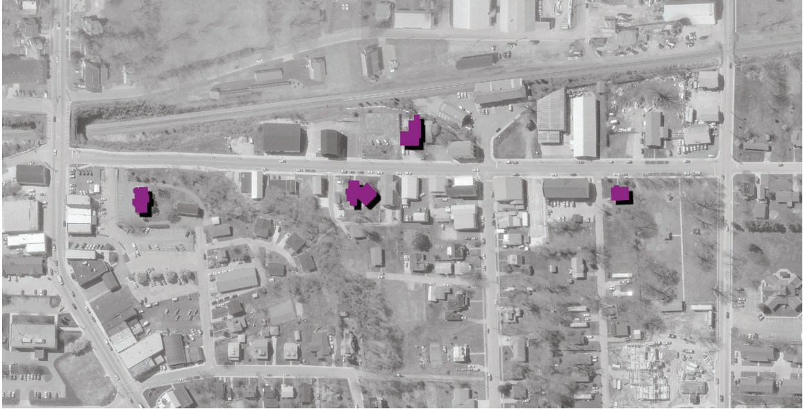
Utilitarian commercial buildings in Old Town are located away from the the intersection of Broadway and Adams Street.
