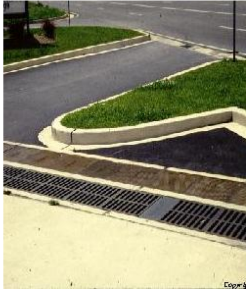
Figure PTP-01- 6 Perimeter Sand Filter
