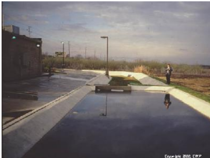
Figure PTP-01- 2 Surface Sand Filter
