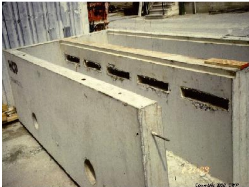
Figure PTP-01- 7 Perimeter Sand Filter
