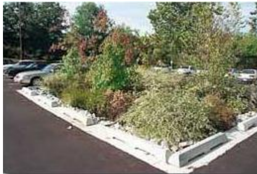
Figure PTP-10- 4 Bioretention System
