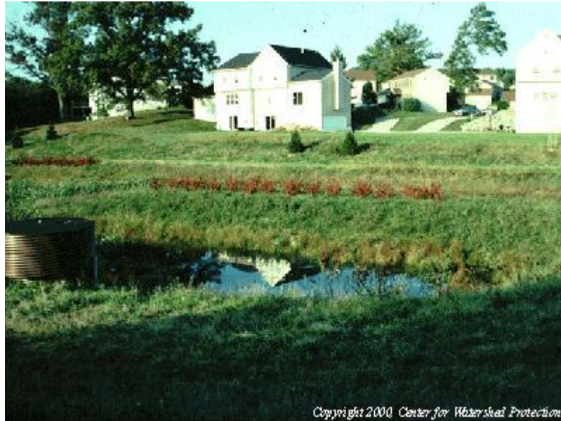
Figure PTP-03- 7 Micropool Extended Detention Pond.
