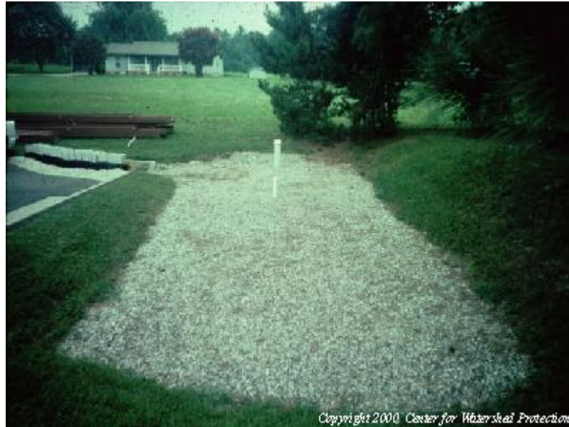
Figure PTP-05- 1 Infiltration Trench
