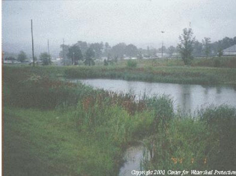
Figure PTP-03- 4 Wet Extended Detention Pond.
