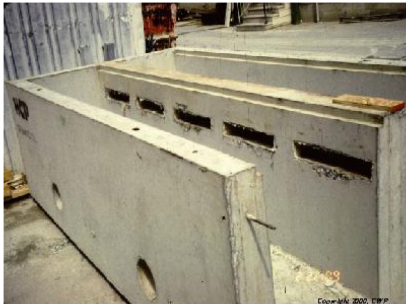
Figure PTP-01- 7 Perimeter Sand Filter
